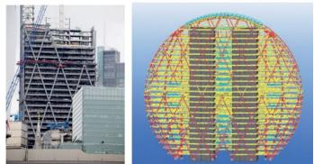
Figure 21. The 14-story module used in The Leadenhall Building in London, England and the 8-story module used in the Aldar Headquarters, Abu Dhabi building (Boake,2014).
