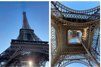
Figure 5. Eiffel Tower, Paris- France, constructed in 1889 with cast iron trusses(Taken by the author, 2020).
