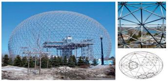
Figure 10. The USA Pavilion designed by Buckminster with a geodesic dome(Silver and McLean, 2013).
