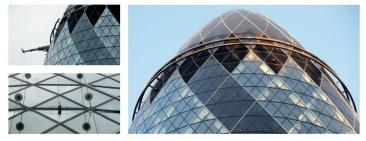
Figure 38. Rail and crane used for facade cleaning of Gherkin Tower(Boake, 2014).
